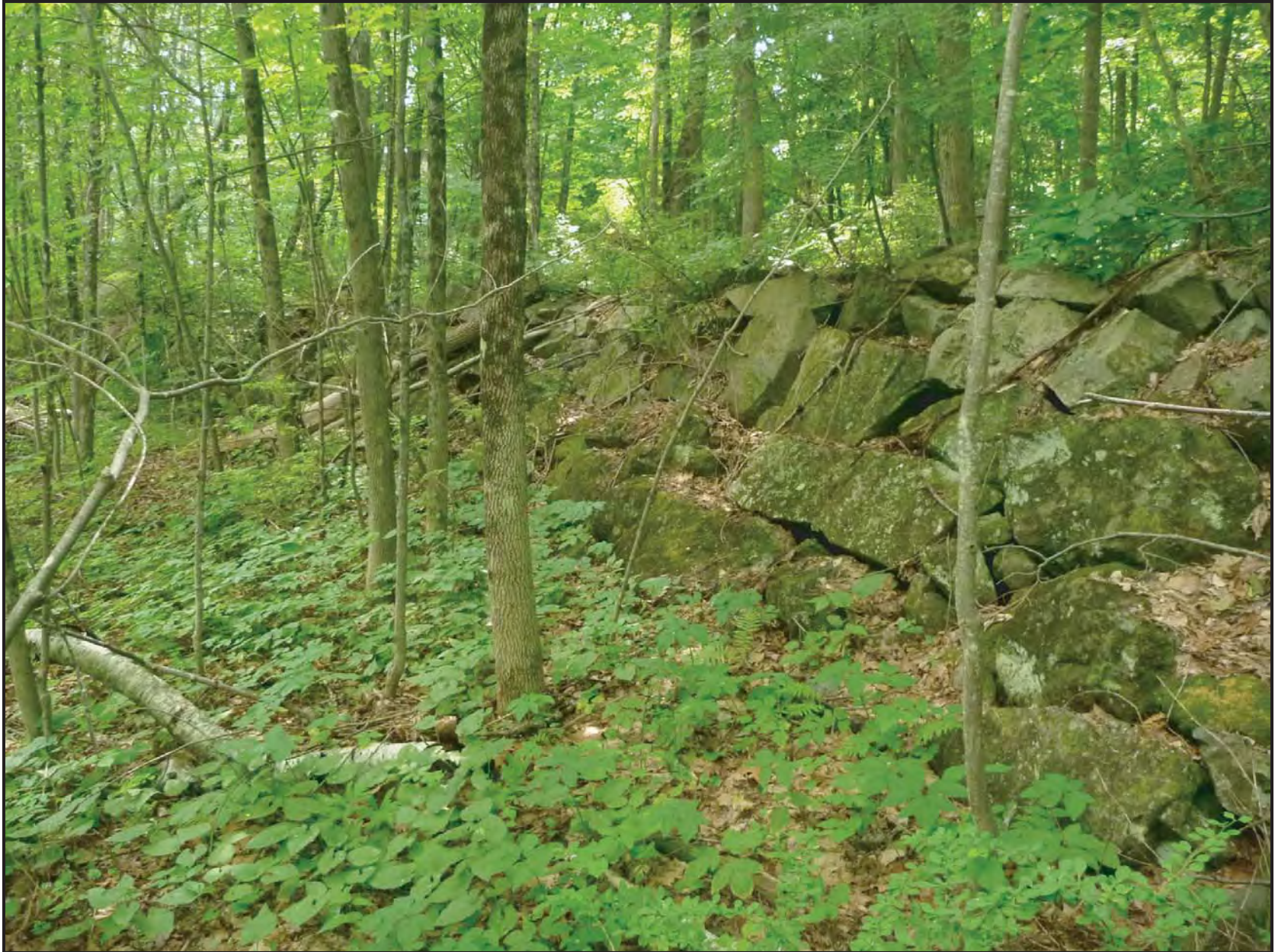
Figure 20. Berm constructed of large granite blocks cuts off the channel's floodplain access immediately upstream of the Main Street bridge in Conway.
