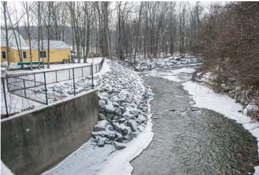
Figure 4. Impact of Tropical Storm Irene flooding and subsequent river management as revealed just upstream of Route 116 Bridge where a) bank repairs completed in early August 2011 were b) washed away by flooding on August 28, 2011 with c) post-flooding bank repairs further constricting channel (photo "c" courtesy of M.Turre).
