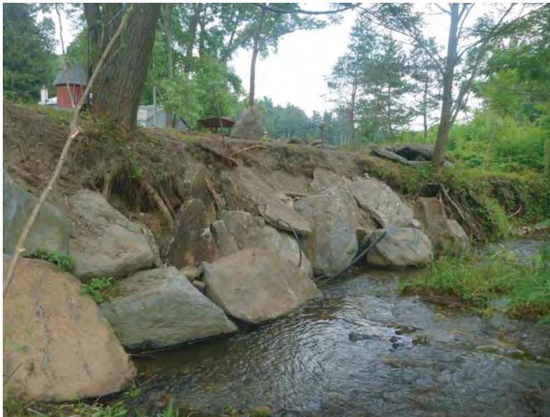
Figure 16. Bank armoring on South River comes in the form of a) concrete retaining walls, b) stacked rock retaining walls and c) rock riprap.
