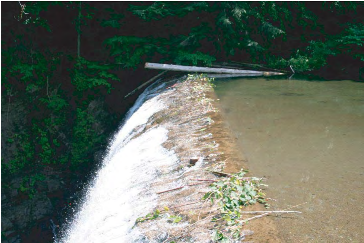
Figure 13. Former dams on South River are a) primarily log crib structures while b) the largest existing dam is made of concrete.
