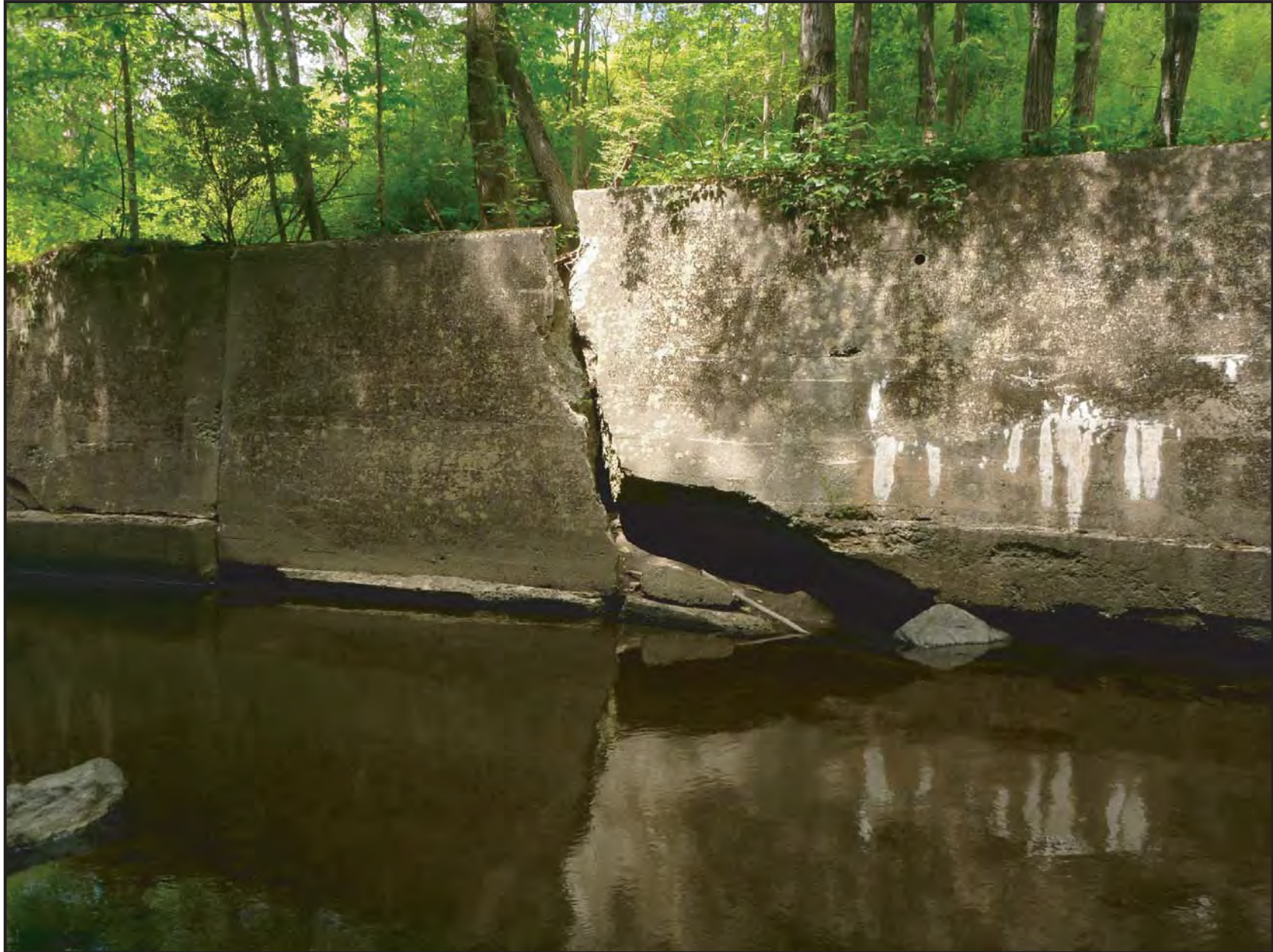
Figure 18. Scour undermines a concrete retaining wall on South River in Conway.
