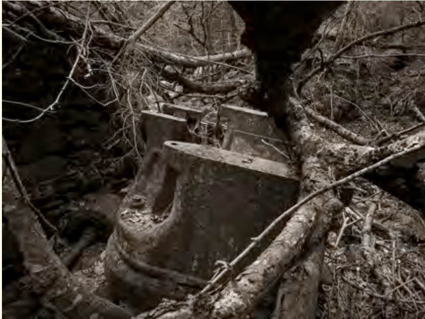
Ruins of generator mount and penstock at the Conway Station dam (Photos by Ben Barnhart, 2012)
