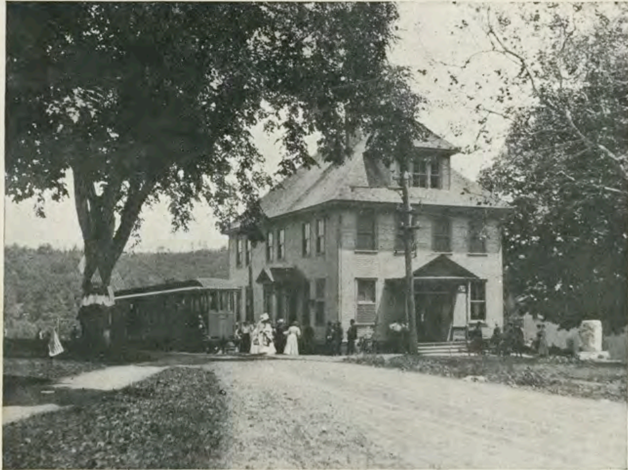
Masonic Building and Electric Station, Conway, Mass.
